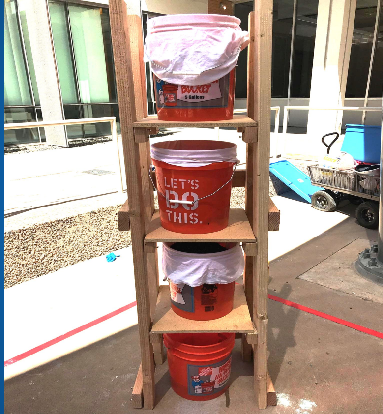
Figure 7: Water Treatment System
